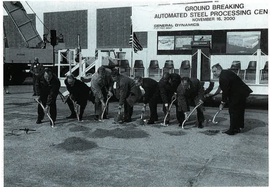
Breaking ground for Quonset Point's $12.4 million automated steel-processing center are from left, John Holmander, site manager; Walter B. Chappel, deputy supervisor of shipbuilding; George Drakeley of the Virginia-class Program Office; John Casey, VP – Operations; U. S. Sen. Jack Reed of Rhode Island; Tom Schumpert, director of the Rhode Island Economic Development Corp.; GD Senior VP John Welch; and EB President Mike Toner.
