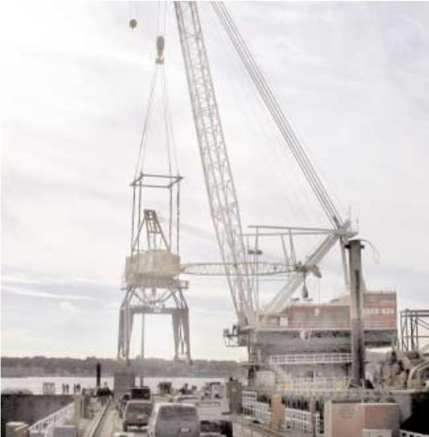
The 75-ton capacity American crane is removed from the North Wall by a 500-ton crane that will transfer it to a support barge. Also removed were the 72-ton capacity "E" Dock American and the 75-ton South Wall Clyde. The two American cranes were taken out of service about five years ago at the completion of the SSN-688 and Trident programs, which they supported. As part of the project, the Center Wall Clyde will move to the South Wall, and a new crane will be installed on the Center Wall.
