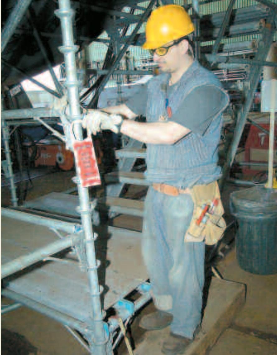
*Carpenter apprentice Tyler King (252) hangs a scaffolding tag on staging in Building 260. The Scafftag system, used on a limited basis for the past three months, will be implemented throughout the Groton shipyard and on EB overhaul and repair projects at the Groton submarine base beginning Sept. 6.*
